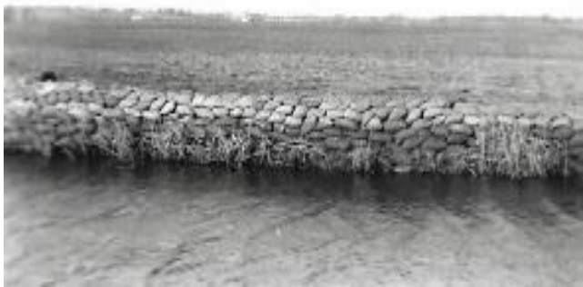
All neatly tidied away
